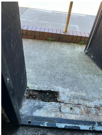
Hole in floor – escape route and damaged handrail
